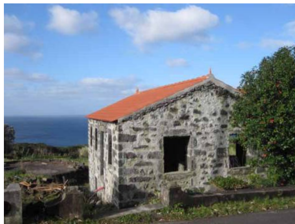
Figure 3: The ruin acquires a roof.
